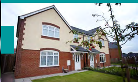
Repairs responsibility P5
